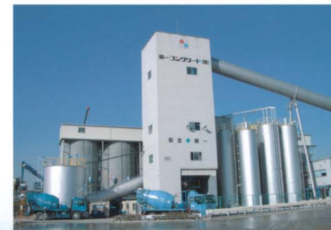
Ready-Mixed Concrete Plant
